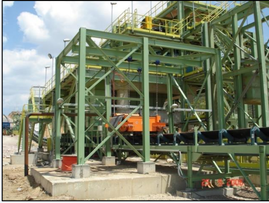
Secondary & Tertiary Crusher
