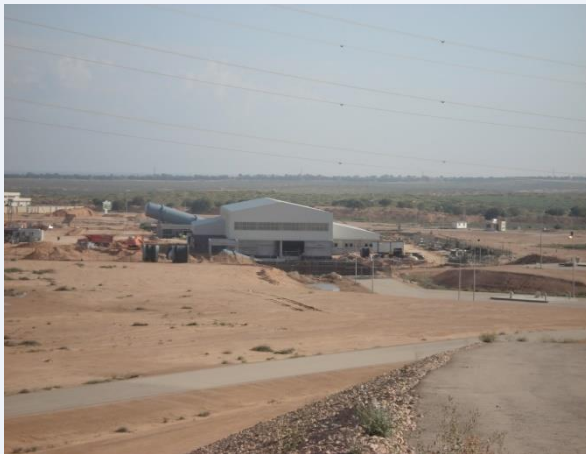
SIRT 'B' Pump Station General View
