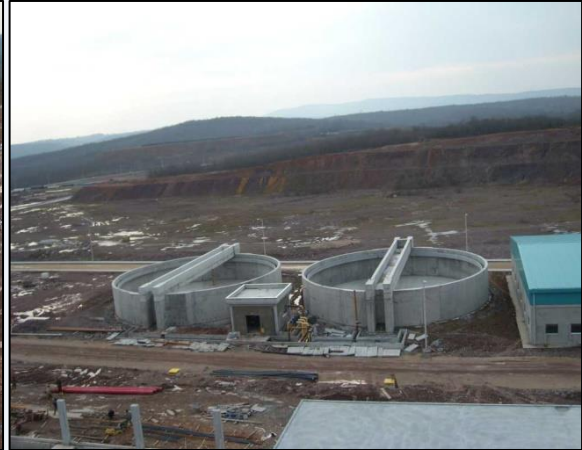
Sludge Thickeners
