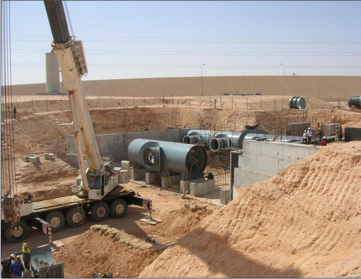
Screen Chamber Construction
